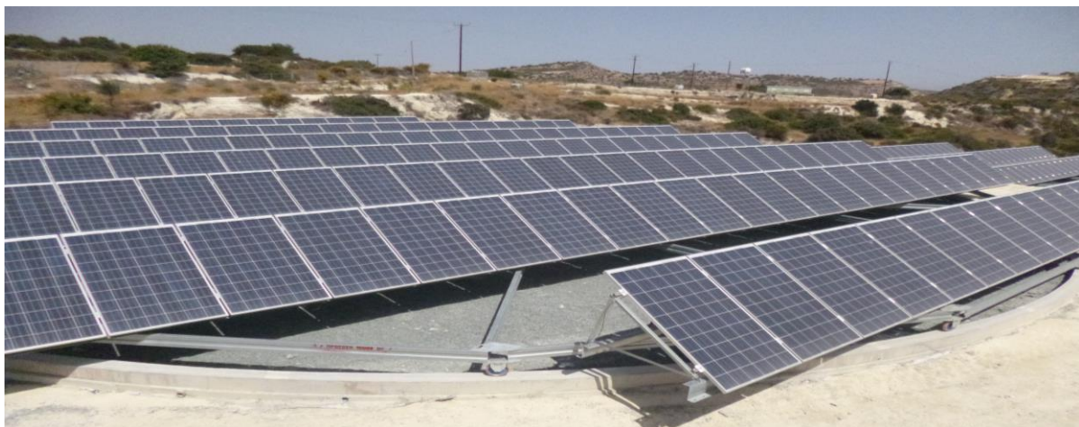
Solar farm in Cyprus, photovoltaic cells are on a rotating platform to track the sun's path.
