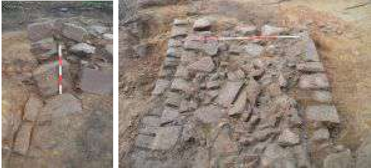
Plate 8: Left. Facing East. North face of Hadrian's wall on cracked foundation slabs. Note the clay and stone revetment (233) supporting the wall on the left to prevent collapse.
